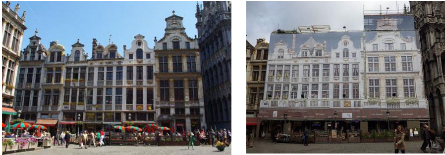
Grand-Place ns 34 to 38, view before and during de restoration.
