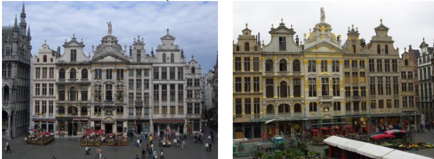
Grand-Place ns 20 to 28, view before and after de restoration.
