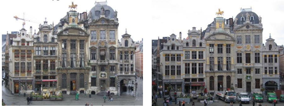
Grand-Place ns 8 to 12, view before and after de restoration.
