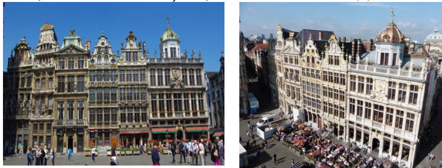
Grand-Place ns 1 to 7, view before and after de restoration.
